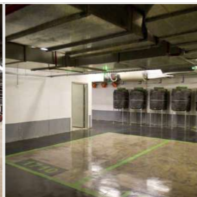
Underground parking in a shelter, Tel Aviv
