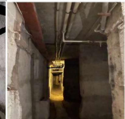
Long basement corridor serving as a shelter
