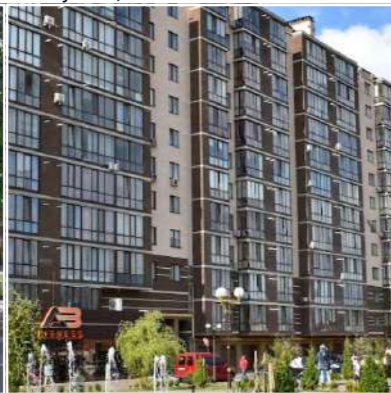
6. Community and Social Amenities (The space around Andora complex)
