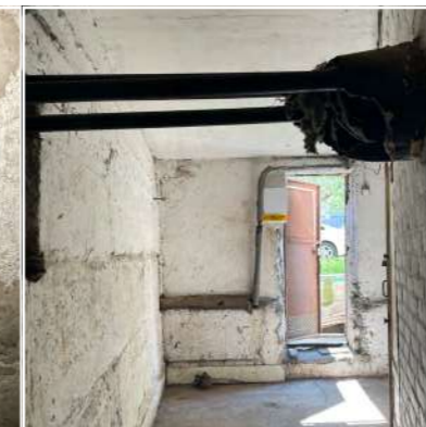
Entrance to the shelter
